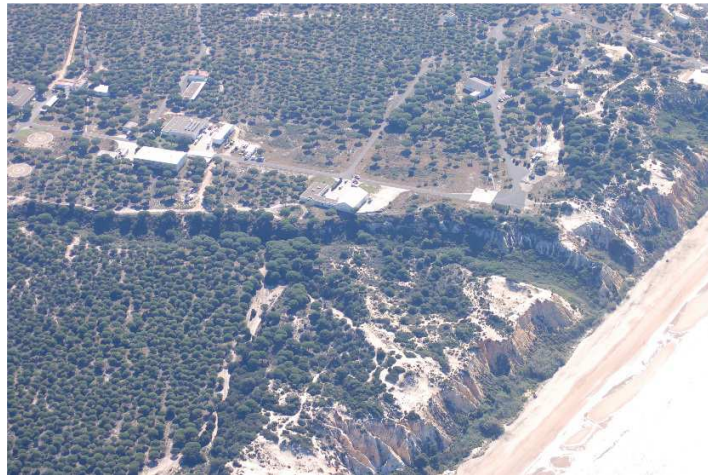
Figure 5. General overview of INTA/CEDEA facilities.
